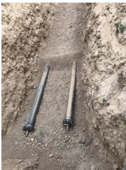
Photo 11: Trench excavation for the water supply network (Chaek Subproject, Chaek Villages (zones #1) Status in November 2024)
