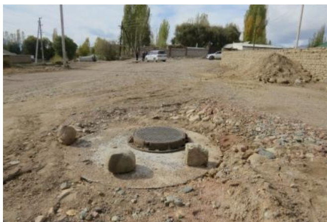
Photo 12: Cast iron hatches were installed on water wells (Chaek Subproject, Chaek Villages (zones #3) Status in November 2024)
