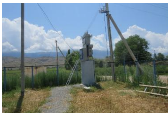
Photo 5: A complete transformer substation (CTS) (Zhan-Bulak Subproject, status: August 2024).
