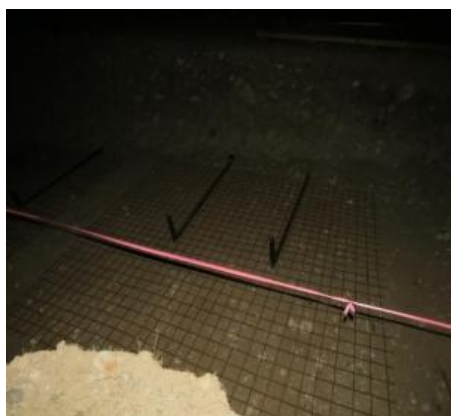
Photo 5: Reonforcement of the reservoir bottom. Photo 6: Drilling the borehole. (Isakeev Subproject, Status in November 2024)
