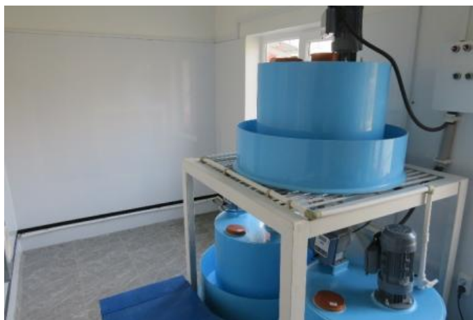
Photo 3: Water disinfection installations with chlorine (1 - working, 1 - backup) (Oruk-Tam Subproject, status: October 2024)
