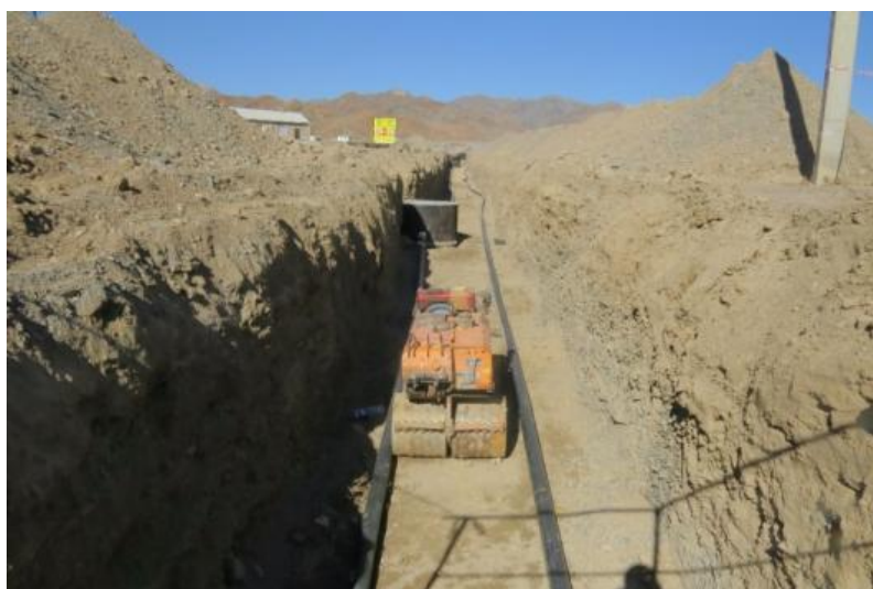
Photo 4: Excavation of the water pipeline trench (Kochkor Subproject, Kara-Too Village, Status in November 2024)
