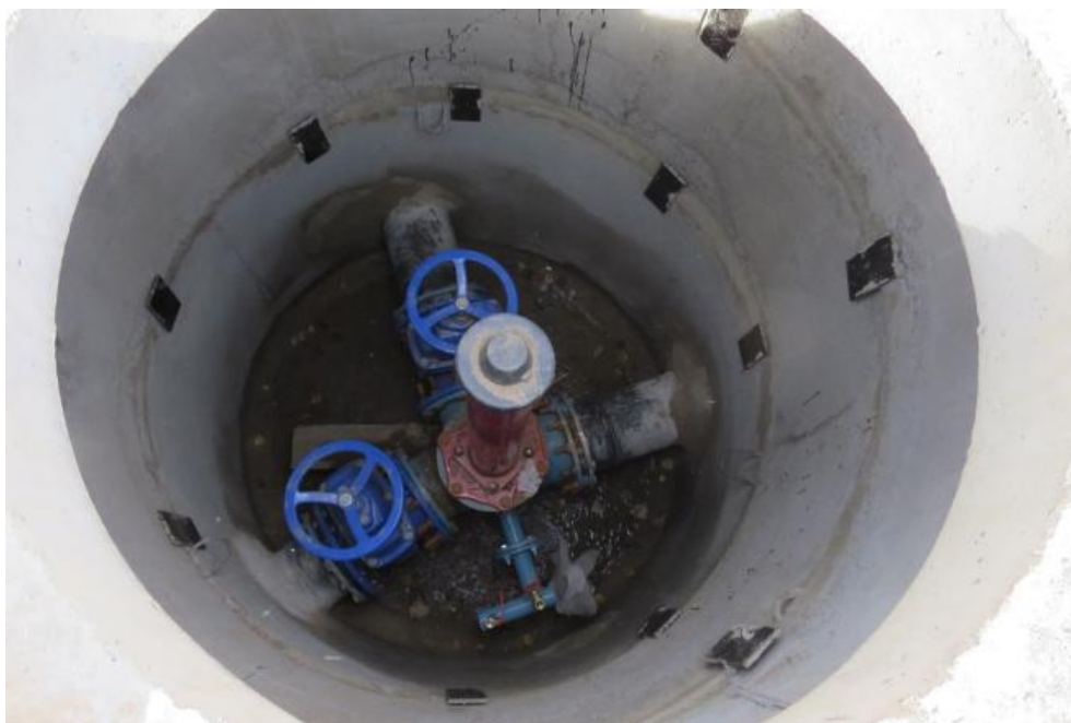
Photo 13: Manifold valves will be installed in water wells and shut-off and control valves (Chaek Subproject, Chaek Village (zone #4) Status in November 2024)
