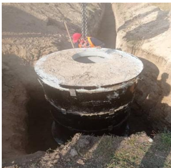
Photo 10: Installation of the well (Lama Subproject, Status in November 2024)
