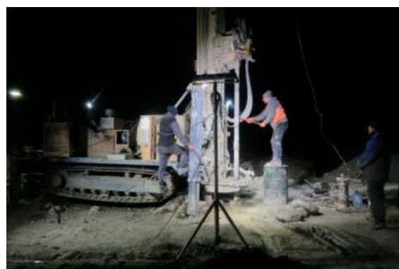
Photo 5: Reonforcement of the reservoir bottom. Photo 6: Drilling the borehole. (Isakeev Subproject, Status in November 2024)
