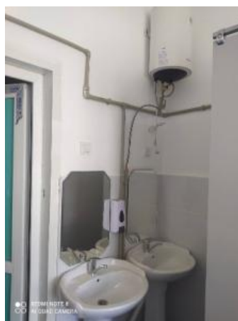
Photo 7: Sanitary devices were connected to hot water (Zhan-Bulak Subproject, school named after A. Zhutakeev, status: August 2024).
