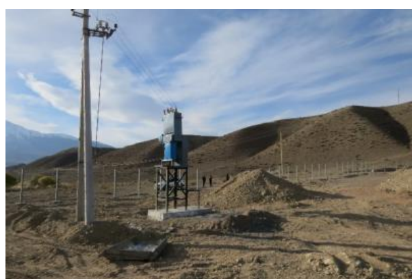
Photo 9: The KTP–25–6–04 was installed
