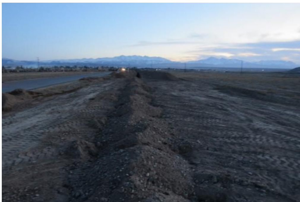
Photo 2: Backfilling the trench (Baetovo Subproject, Kaindy-Bulak Village, Status in October 2024)
