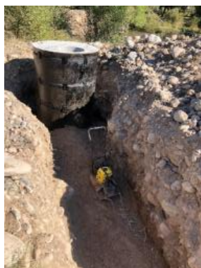
Photo 7: Excavation of water supply network trench and installation of wells (Moldo-Kylych Subproject, Status in November 2024)
