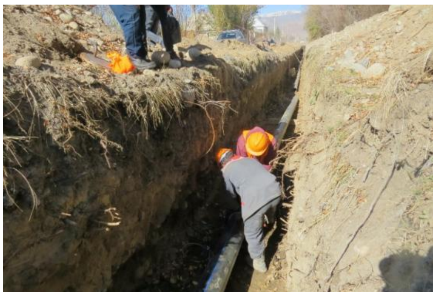
Photo 3: Excavation of trench for a water supply network (Kochkor Subproject, Kochkor Village, Status in November 2024)
