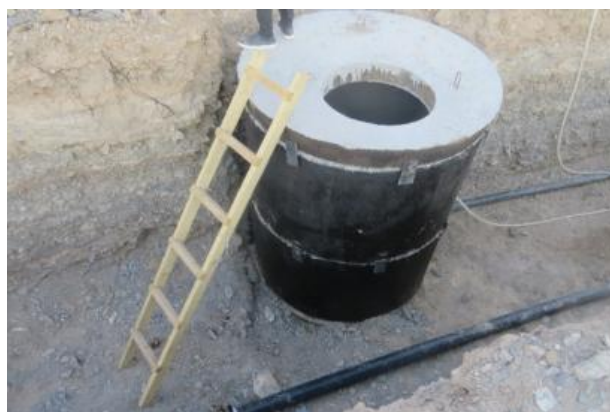
Photo 18: Installed temporary ladders for construction and installation work (Moldo-Kylych Subproject, Status in November 2024)
