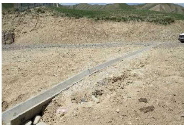
Photo 11. Through mudflow drainage structures in order to protect against floods and mudflows (Tosh-Bulak Subproject, status: May 2024).
