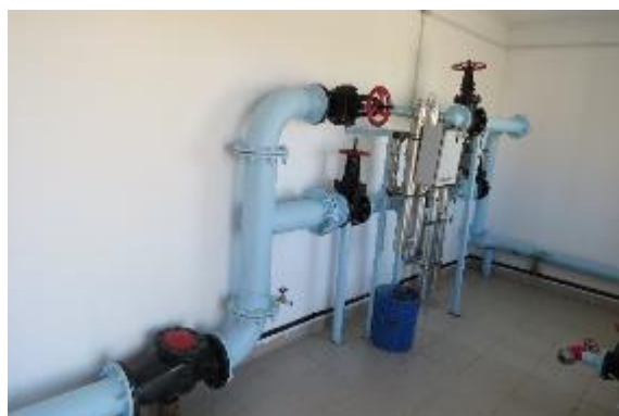
Photo 4. Bactericidal installations in the amount of 2 pieces, located in the technical room (Zhan-Bulak Subproject, Status in May 2024)
