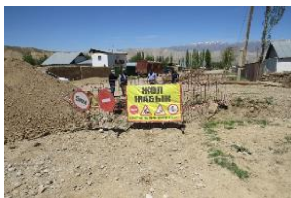
Photo 15. In the populated area, protective fences were installed along the perimeter of the trenches and Warning Signs (Zherge-Tal Subproject, Status in May 2024)
