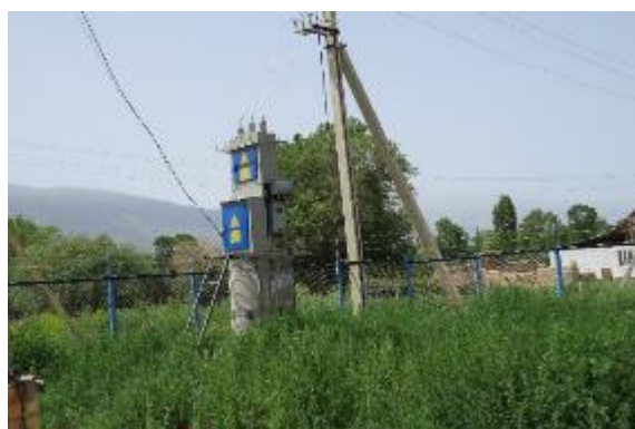
Photo 2. The complete transformer substation (CTS) (Zhan-Bulak Subproject, Status in June 2024)
