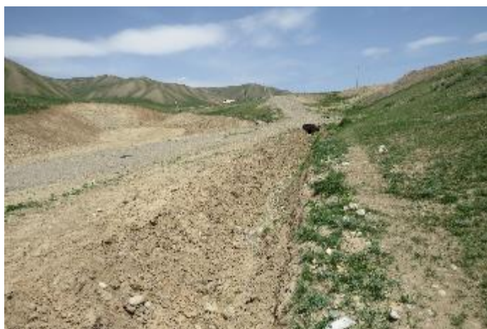
Photo 10. Earth mudflow drainage structure in order to protect against floods and mudflows (Tosh-Bulak Subproject, status: May 2024).
