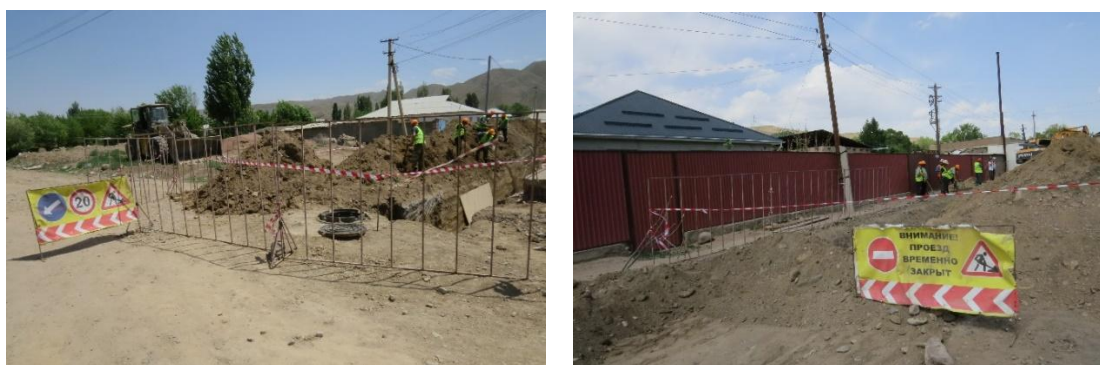
Photos 9–10: Reflective warning signs and fences have been installed on the trenches (Chaek village (Zone #1), status: May 2025)
