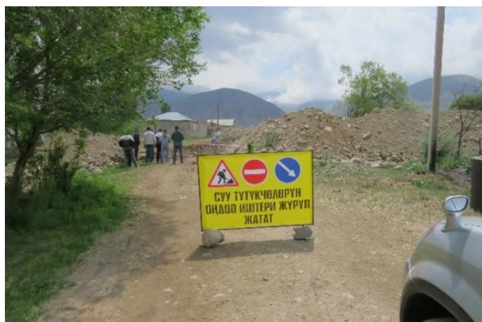
Photo 30: Installed Warning Signs (Isakeev Subproject, Status in June 2025)
