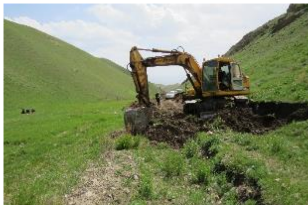
Photos 1–2: Construction of the road to the water supply source. Excavation of water pipeline trench (Lama village, status: May 2025)
