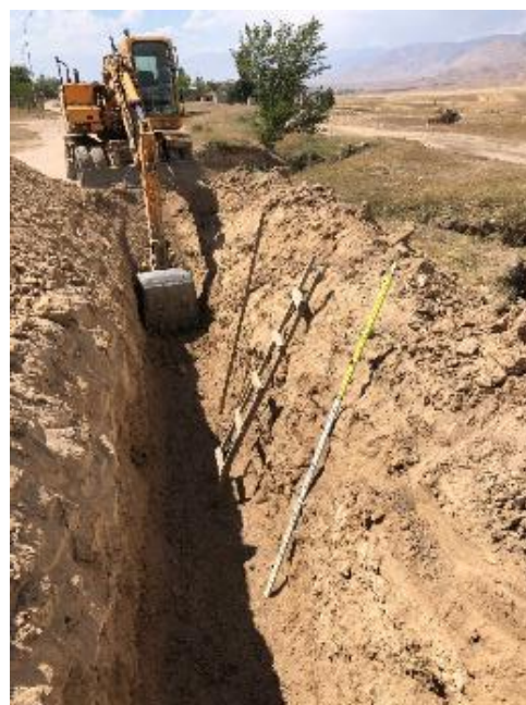
Photos 1–2: Construction of the road to the water supply source. Excavation of water pipeline trench (Lama village, status: May 2025)
