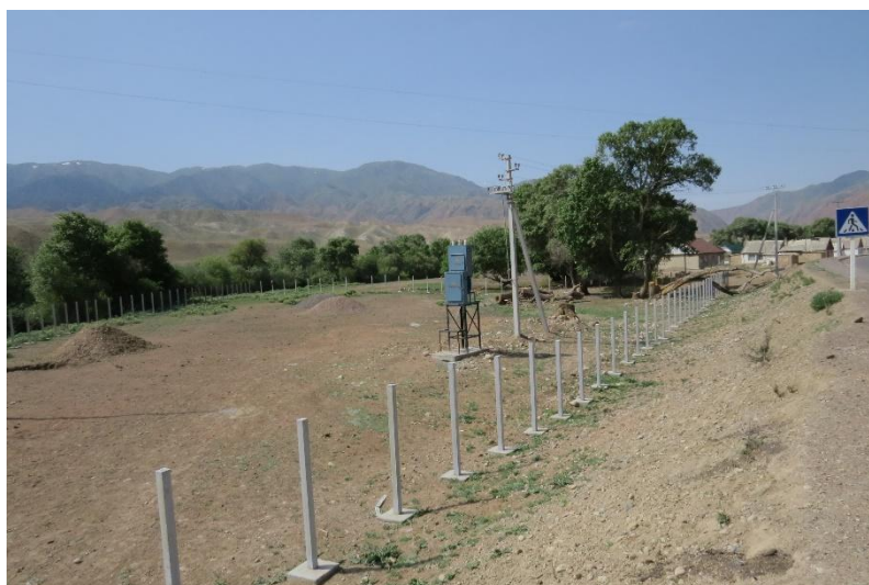
Photo 41: Posts have been installed to fence off the water intake area (Aral Subproject, Status in June 2025)
