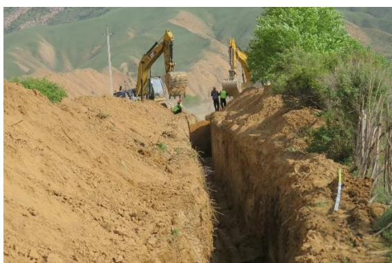
Photos 25–26: Laying the water pipeline from PE pipes. Inspection of the water supply source (Kulanak village, status: May 2025)
