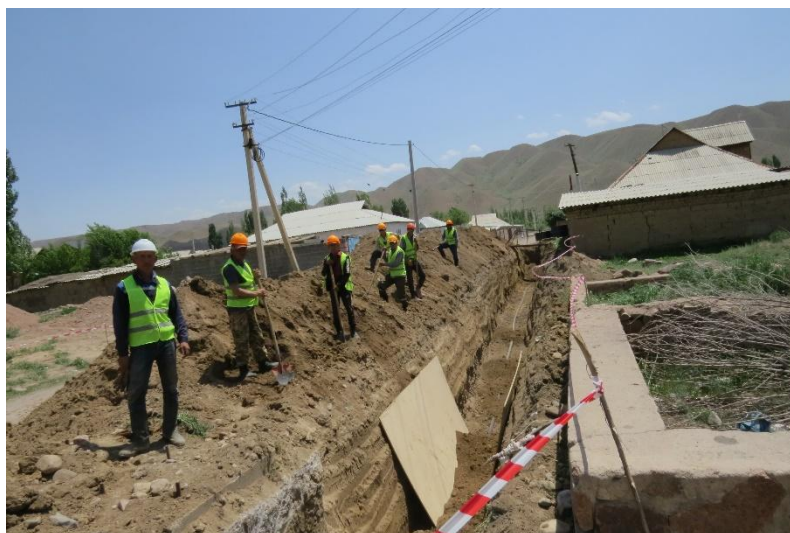
Photo 36: Workers have been provided with special clothing and personal protective equipment (PPE) (Chaek Subproject, Status in June 2025)
