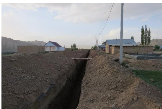
Photos 23–24: Temporary crossing bridges have been installed on the trenches. The village roads have been restored (Kaiyndy-Bulak village, status: May 2025)
