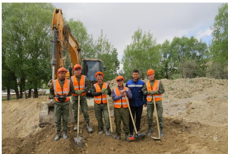
Photo 35: Workers have been provided with special clothing and personal protective equipment (PPE) (Zherge-Tal Subproject, Status in June 2025)
