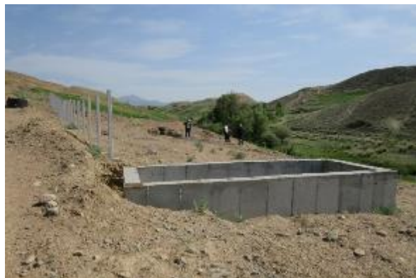
Photos 5–6: Spring catchment chambers. Reservoir site (Besh-Terek village, status: May 2025)
