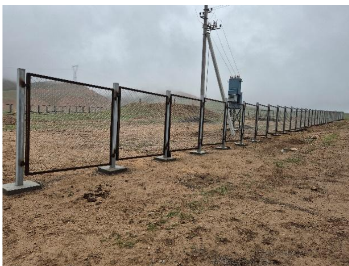
Photo 29: The reservoir site is completely fenced (Lama Subproject, Status in June 2025)
