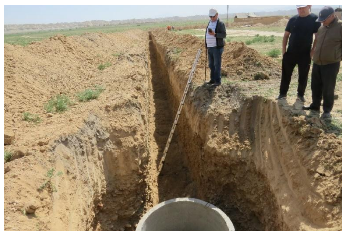
Photo 31: Installed temporary ladders for construction and installation work (Baetov Subproject, Status in June 2025)
