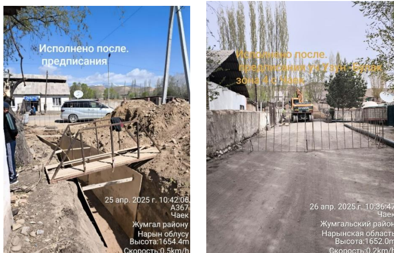
Photos 7–8: Excavation of water pipeline trench (Chaek Village (Zone # 4), status: April 2025)
