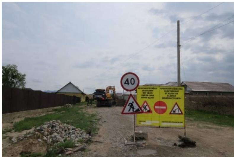
Photo 42: Reflective signs were installed (Kochkor Village, Status in June 2025)
