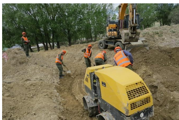
Photos 27–28: Compaction after laying the water pipeline. Contractor's banner (Zherge-Tal village, status: May 2025)
