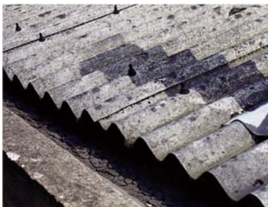
AC sheets used as roofing
