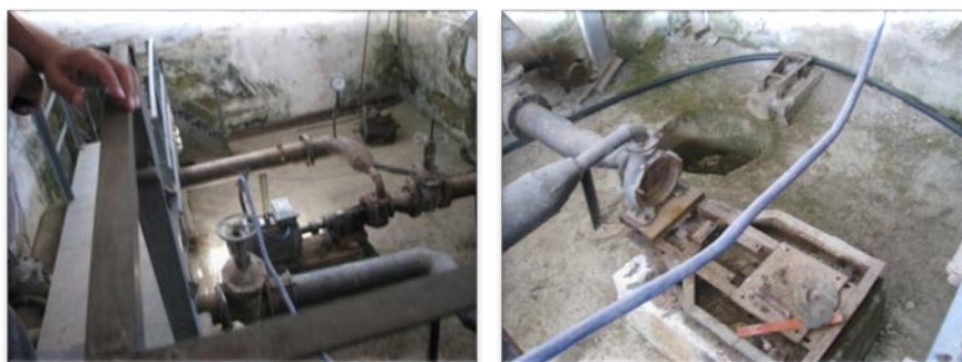
Picture 1-2. Current condition of pumping stations at water intake "Zapadnyi"
