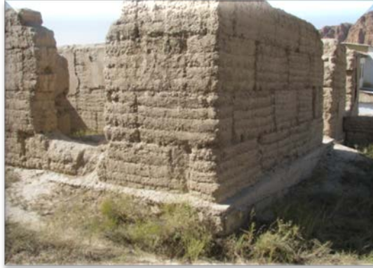
Picture 7. Partially constructed structure on the area of the plot No. 172 in Asko-Too str.
